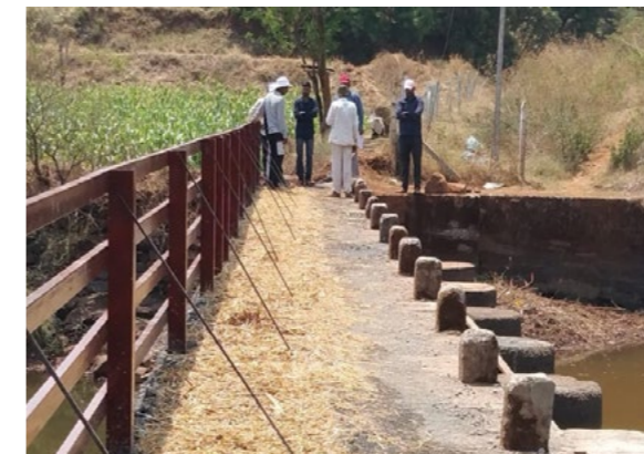
Check Dam Repair
