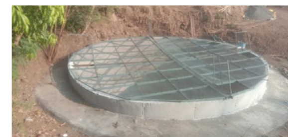
Andgaon Open Well
