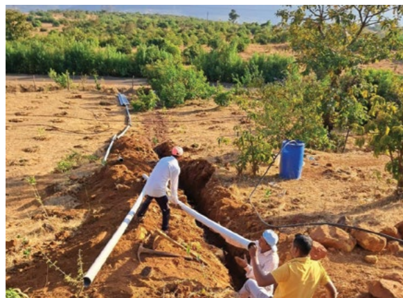
Pipeline Laying for Water Arrangements
